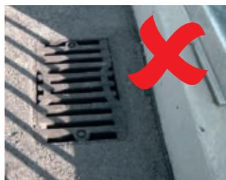
**Fig. 1** Positioning the bridge gully 100 mm from the curb
