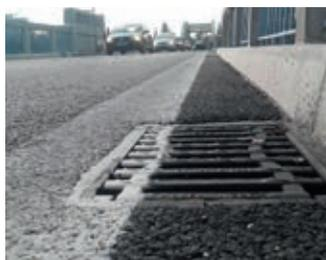
**Fig. 2** Positioning the bridge gully right at the curb
