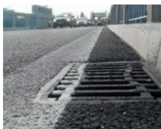
**Fig. 2** Positioning the bridge gully right at the curb
